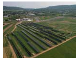
Solar Field (AES)
