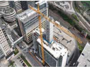
3600 Civic Center Boulevard
